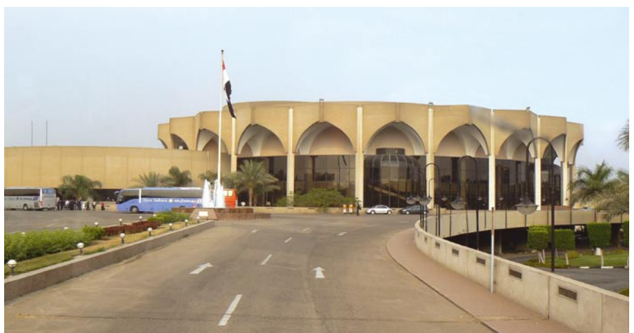
Cairo International Conference Centre (outside). Photo P. Hellström.
